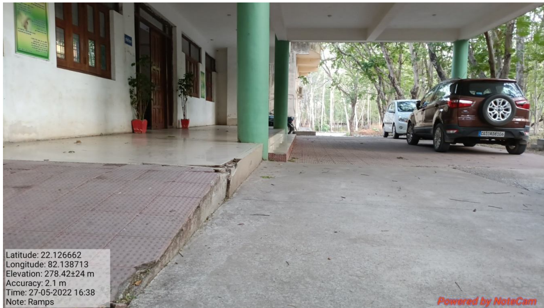
Ramp –Department of Forestry
