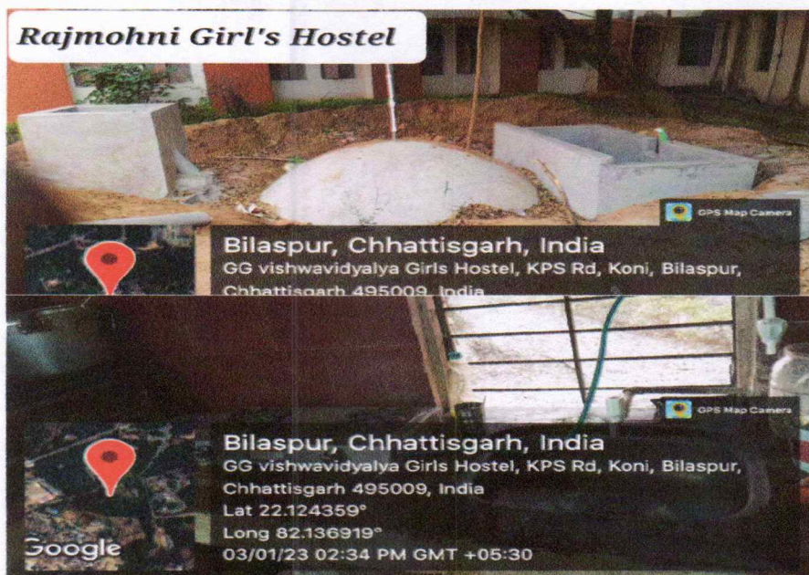
BIOGAS PLANT IN CAMPUS
