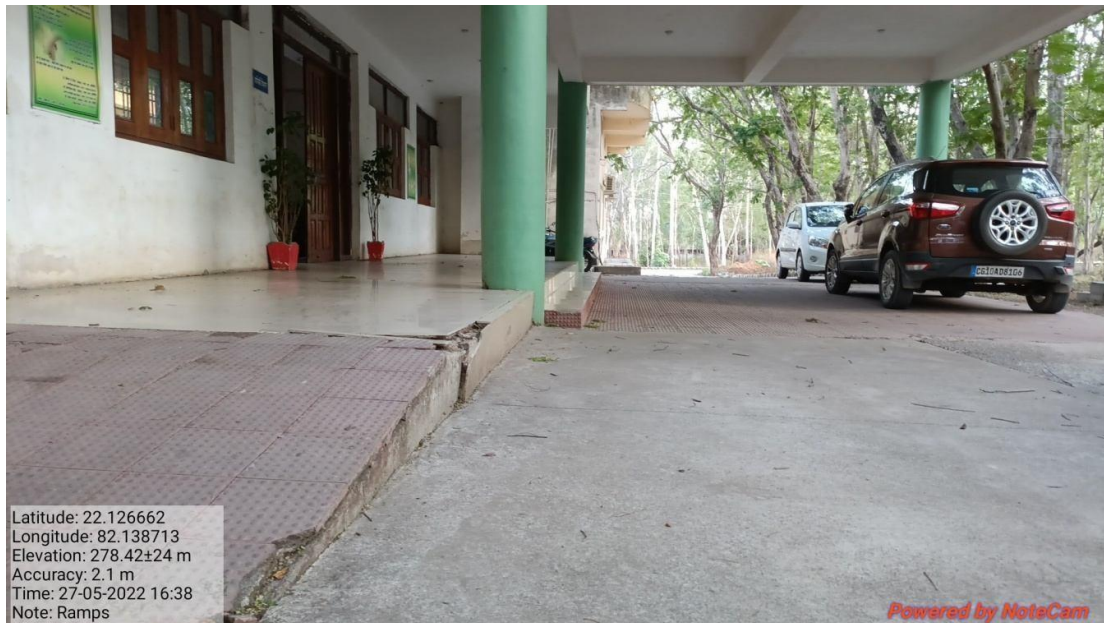
Ramp – Department of Forestry
